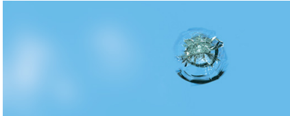
Cracked glass (equal to or more than 1 cm in diameter) or spidered cracks
