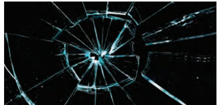
Cracked glass (equal to or more than 1/2" in diameter) or spidered cracks
